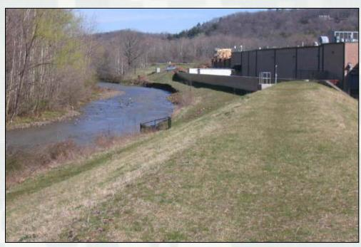
Floodwall & Raised Ground Surface (grass berm with interior floodwall)
