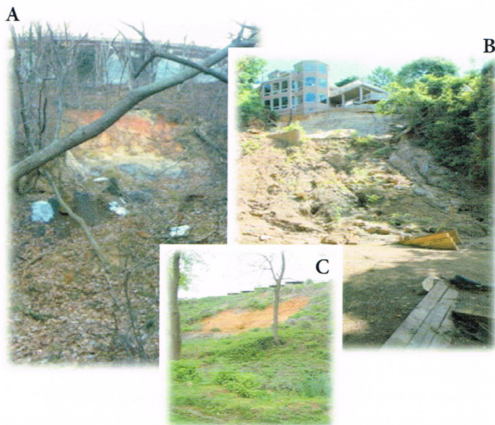
Figure 1. Photographs of three recent shallow landslides in Atlantic Highlands, NJ; A. May 2012 landslide, B. April 2014 landslide, C. One of three landslides in Highlands that occurred during Tropical Storm Irene in August 2011.
