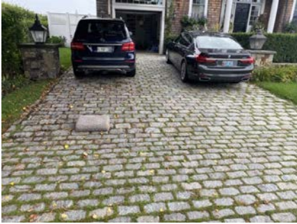
Porous paving in a driveway
