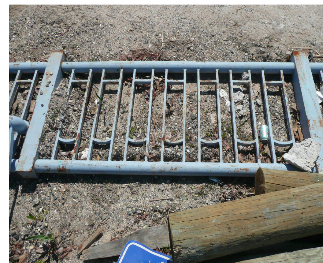
PHOTO OF EXISTING RAILINGS
