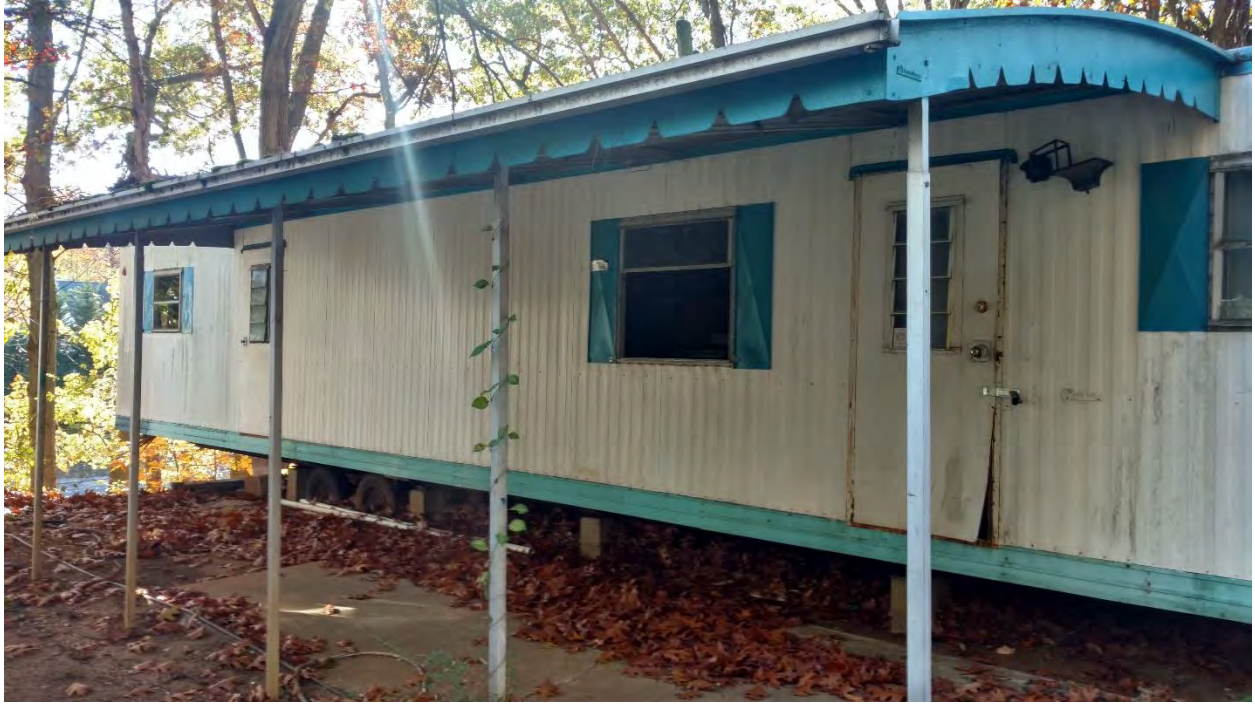
Uninhabited trailer with broken out windows and no steps. The rear portion is over the slope.
