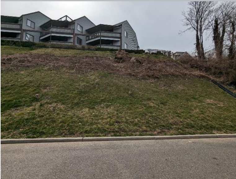
VERY STEEP (BETWEEN 55% AND 70% SLOPE), ERODED SLOPE OR TURF-COVERED SLOPE
