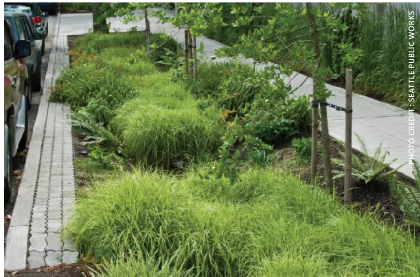
MAINTENANCE STRIP AND CURB CUTS AT STORMWATER PLANTER
